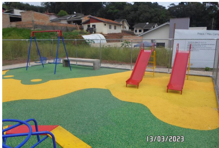
Figure 4 - Piso emborrachado instalado
