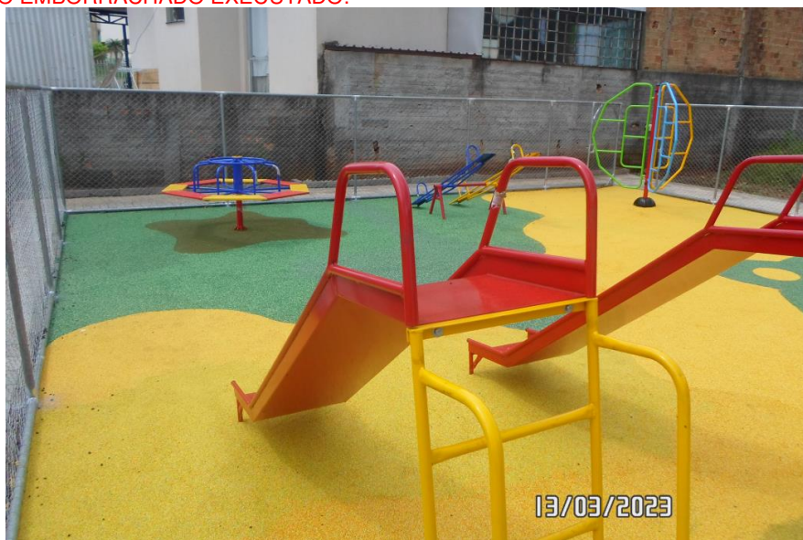
Figure 3 - Piso Emborrachado instalado
